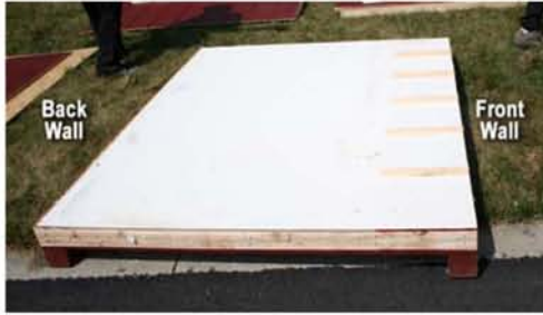
Floor with Nest Box Dividers NOTE: Glasbord flooring attached
