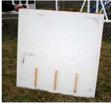
Floor with Nest Box Dividers NOTE: Glasbord flooring attached
